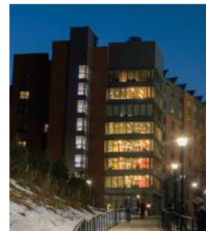
Werth Residence Hall
