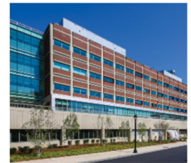
Gant Building Renovation Phase II
